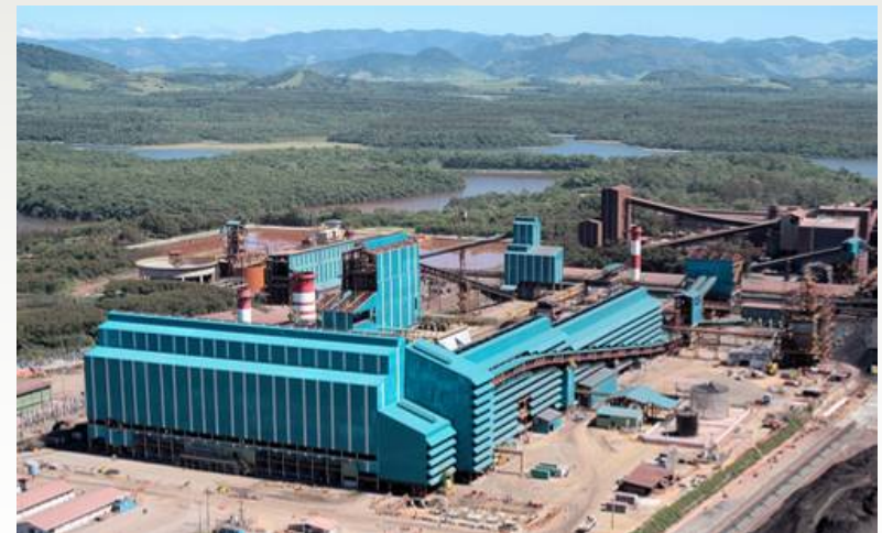
Above: New stacker and reclaimer at Area C operating at design rates Below: Samarco pellet plant 3
