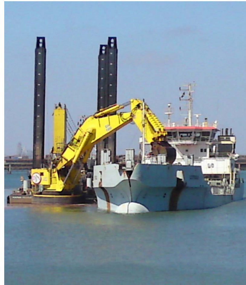
RGP6 dredging work underway at Port Hedland
