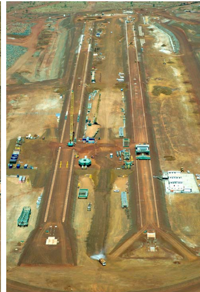
RGP5 Yandi stockyard construction December 09
