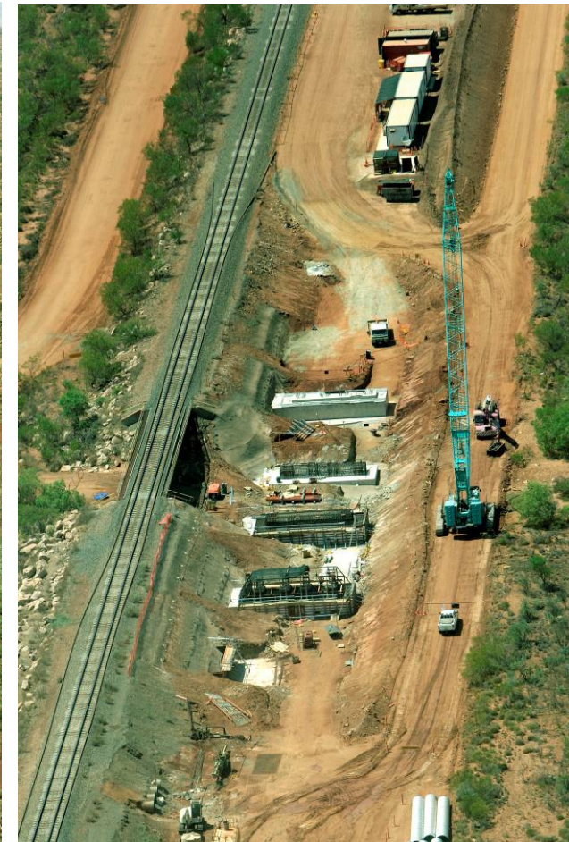
Bore Creek bridge construction, December 2009
