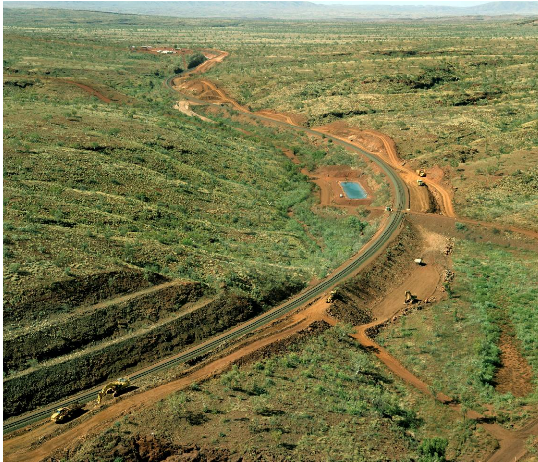
Rail duplication underway Kurrajura to Yandi, December 2009
