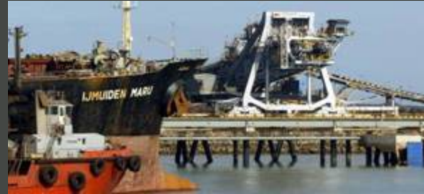
New record loading rate for three shiploaders at Port Hedland
