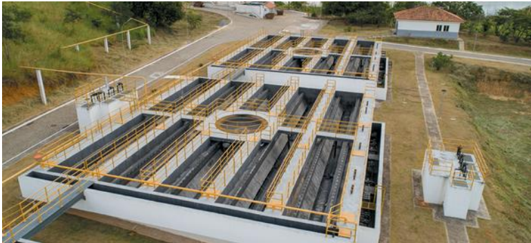
Sewage treatment plant, Colatina
