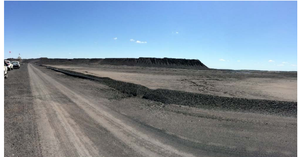
Goonyella Tailings Storage Facility, BMA Queensland Australia
